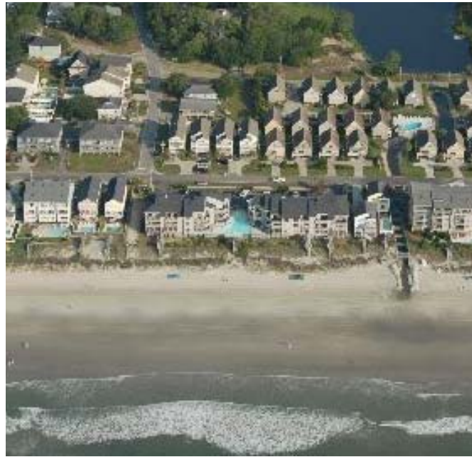
Figure 36. Aerial photograph of northern Surfside Beach. (Photo Credit Scott Harris, June 22, 2007)
