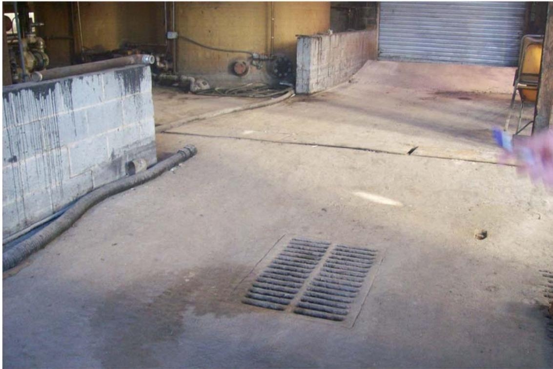
**Photo 11:** Storm water catch basin for the underground cistern located outside the northeastern portion of the mill building at the emulsion plant.
