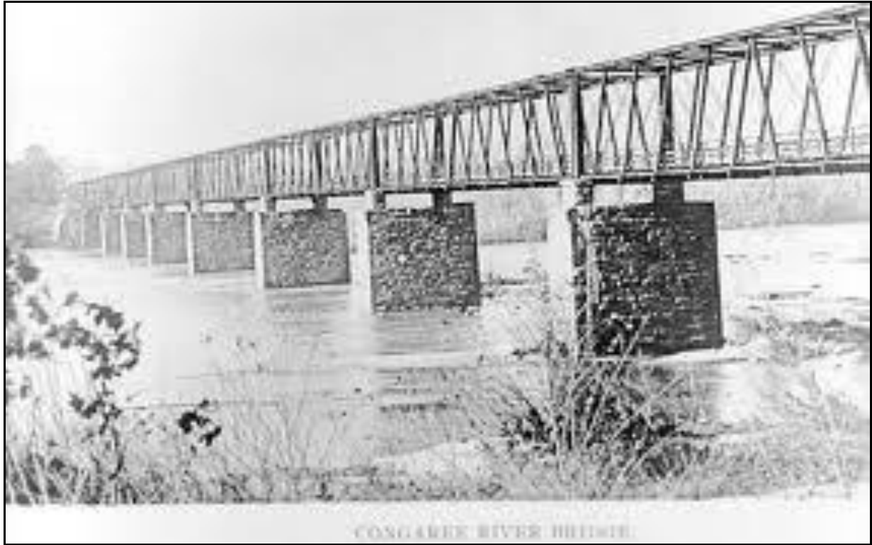
Figure 18. Previous Gervais Street Bridge circa 1900 (photo courtesy of the Carolina Library).
