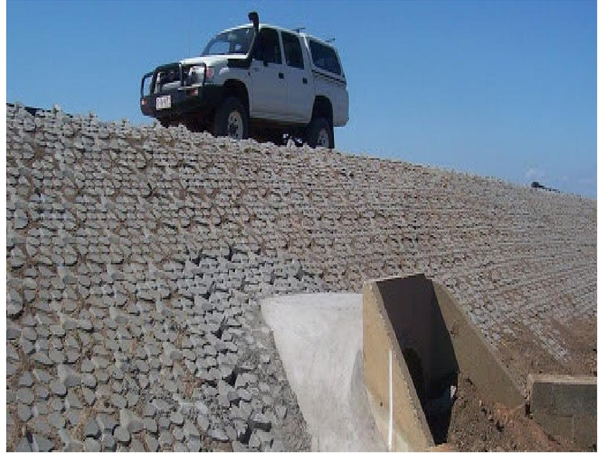
Examples of articulated concrete block mats that will be used to reinforce the rockfill cofferdam on sides and top.
