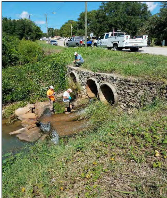
Memorial Park Outfall - SW-01 (Typical)
