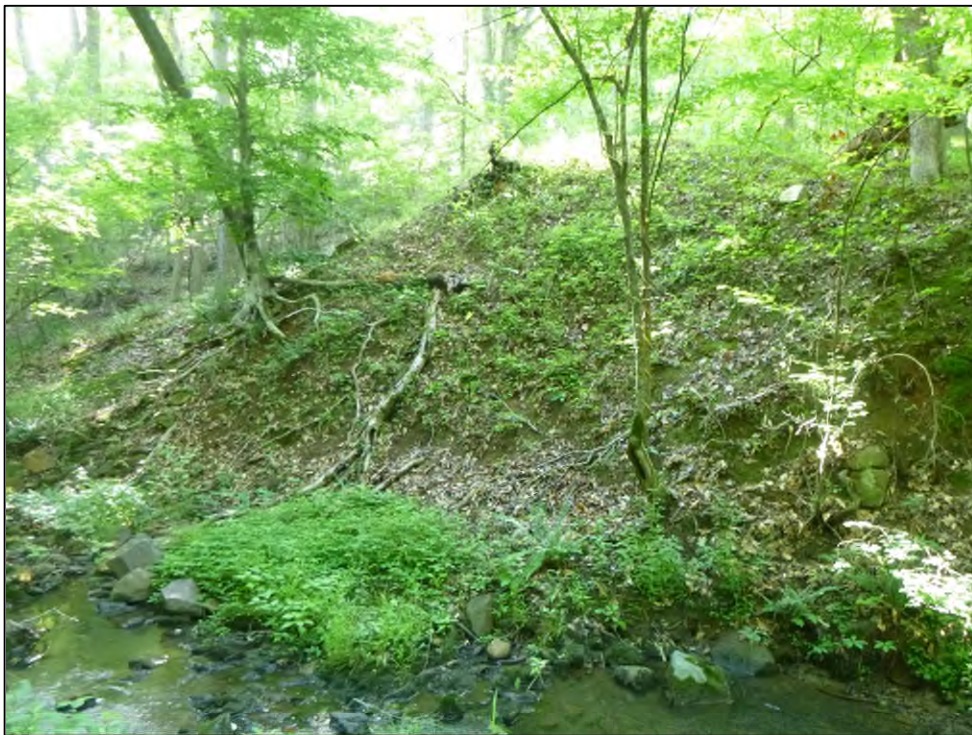
Figure 5.55. One side of the earthen dam at site 38FA675, facing west.
