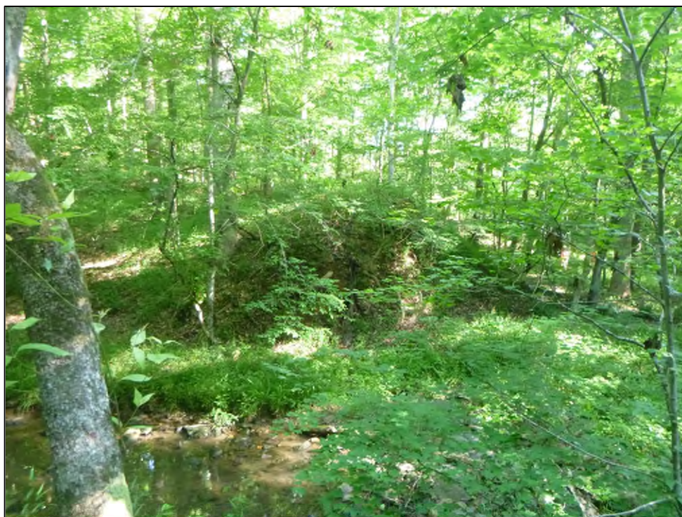
Figure 5.56. One side of the earthen dam at site 38FA675, facing west.
