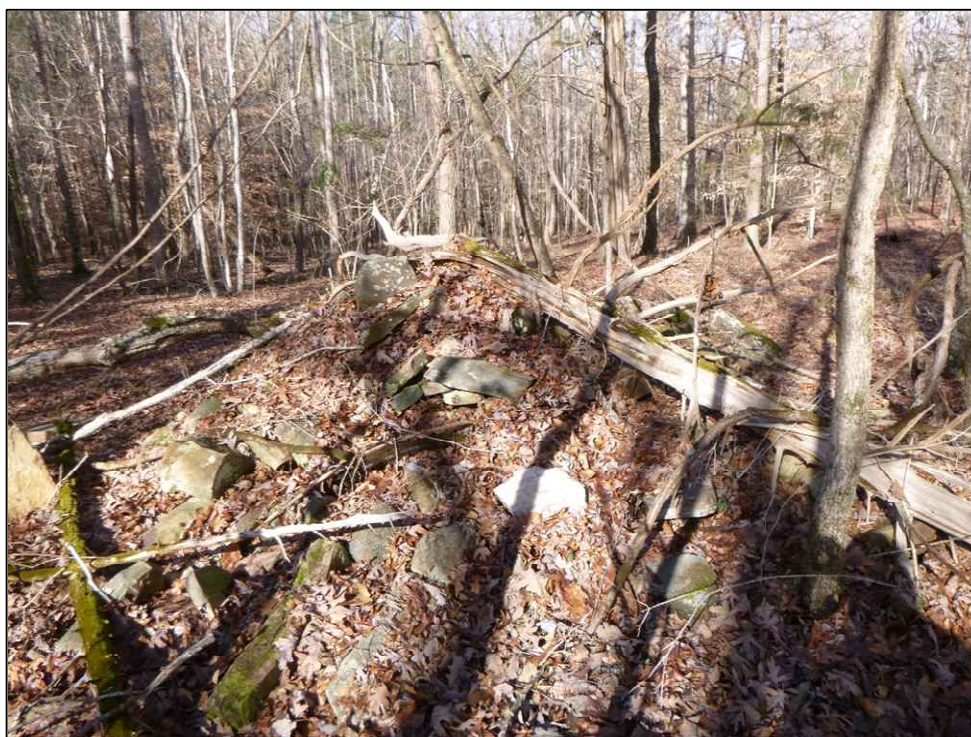
Figure 5.24. View of collapsed fieldstone chimney at site 38FA667, facing west.
