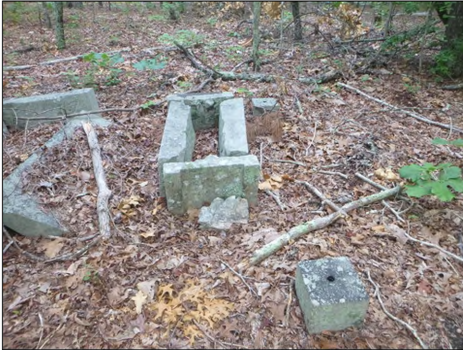
Figure 5.85. Damaged crypt in Old Homer Baptist Church Cemetery (SHPO Survey Number 0113; Site 38FA670).
