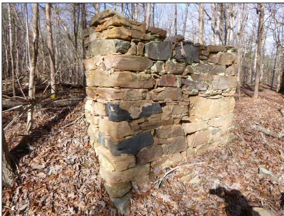
Figure 5.26. View of fieldstone chimney base at site 38FA667 in early 2021, facing northwest.
