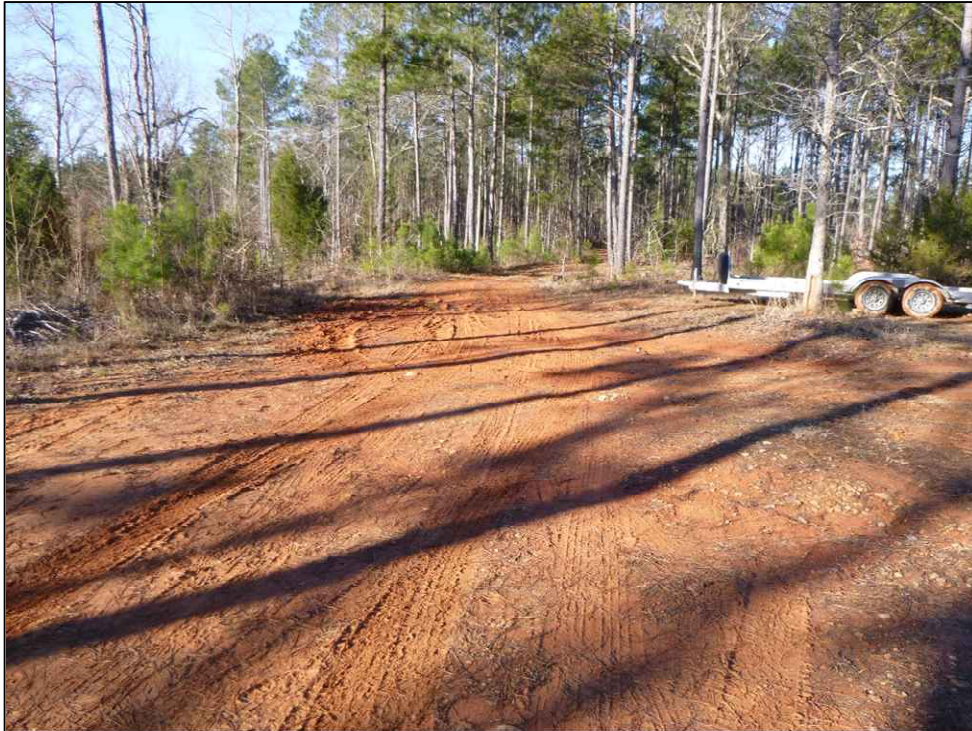
Figure 5.5. Typical dirt road within the project area, facing southwest.
