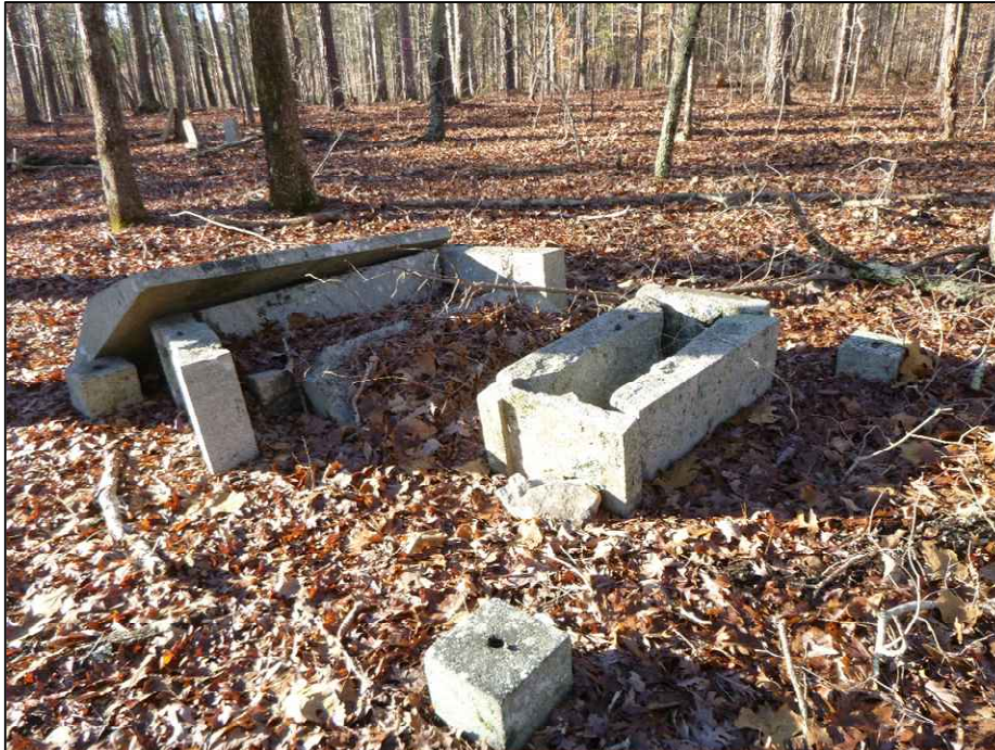
Figure 5.73. Crypts in the Old Homer Baptist Church Cemetery (SHPO Survey Number 0113; Site 38FA670), facing west.
