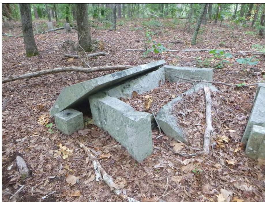
Figure 5.84. Damaged crypt in Old Homer Baptist Church Cemetery (SHPO Survey Number 0113; Site 38FA670).
