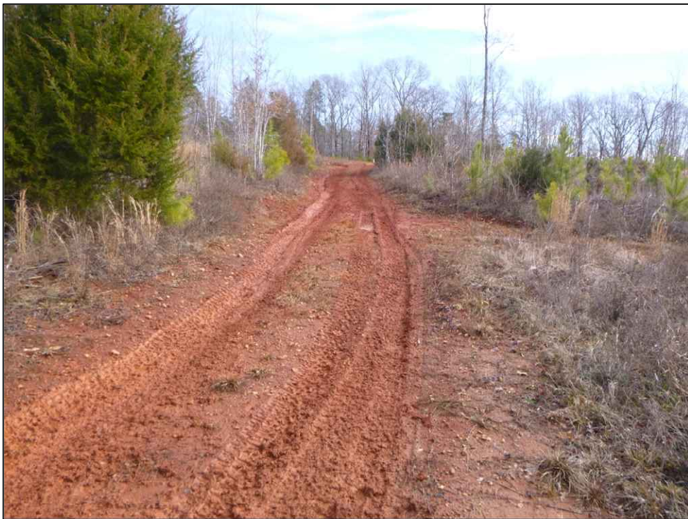
Figure 2.6. Typical dirt road within the project area, facing east.
