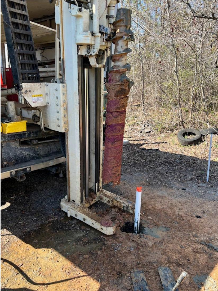
*A groundwater monitoring well being installed at the I-85 Distribution Center site. Total costs of the site for FY22 were approximately \$64,218.*
