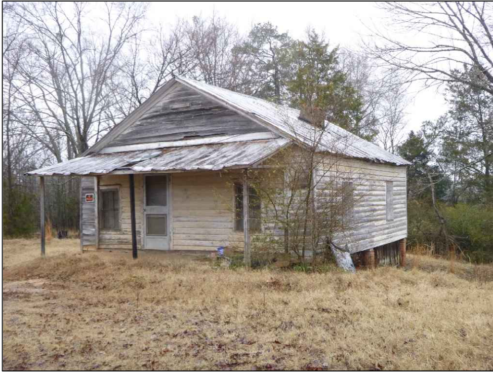
Figure 5.22. SHPO Survey Number 1460, facing north.
