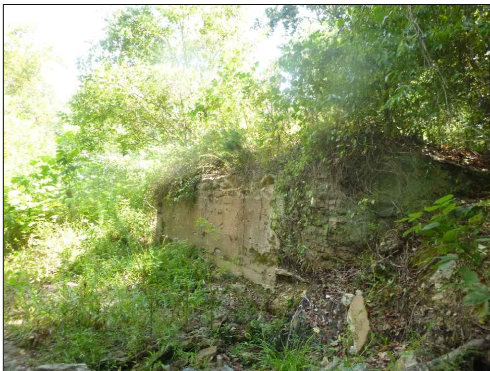
Figure 5.24. Hannah Creek Bridge Abutment (1455), facing southeast.
