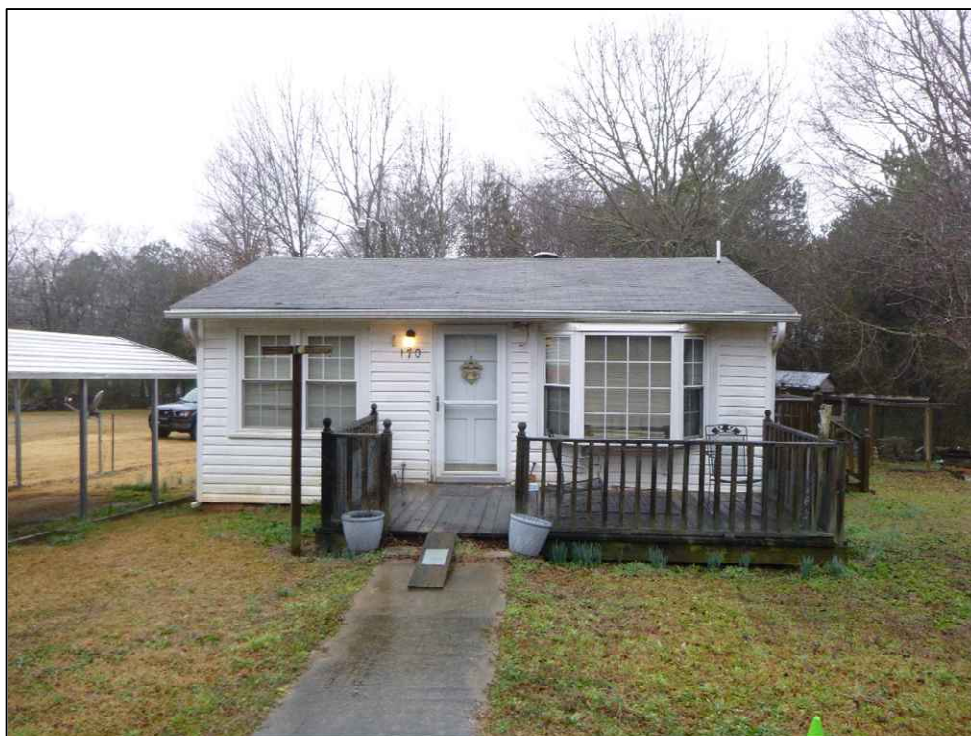
Figure 5.28. SHPO Survey Number 1652, facing north.
