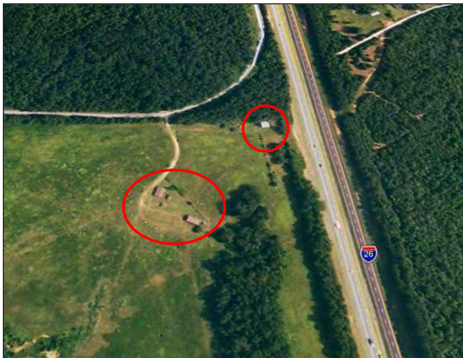
Figure 5.18. Google Earth imagery from 2005 showing buildings in the project area.
