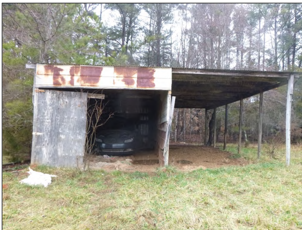
Figure 5.11. Barn/garage in the northern parcel, facing east.
