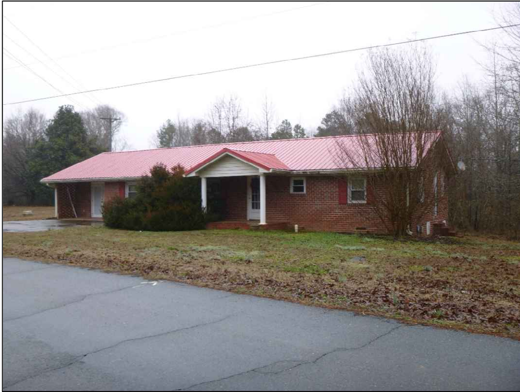
Figure 5.38. SHPO Survey Number 1662, facing east.
