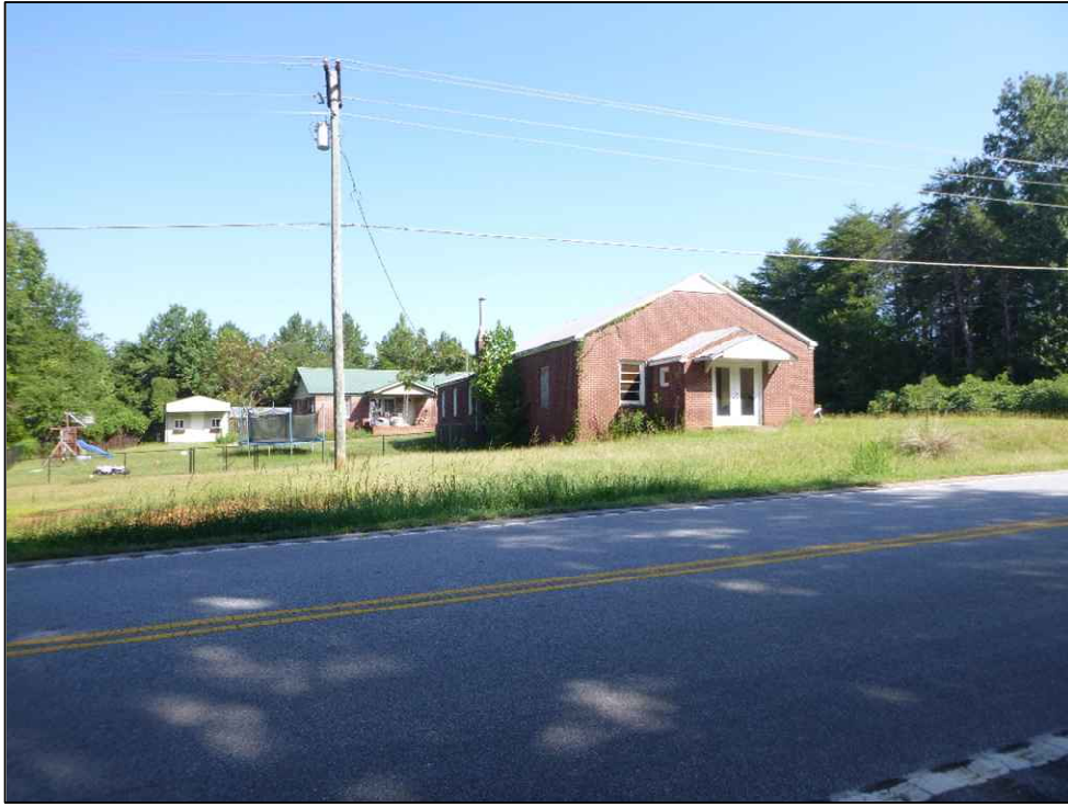
Figure 5.34. Structure 1462, facing northeast.
