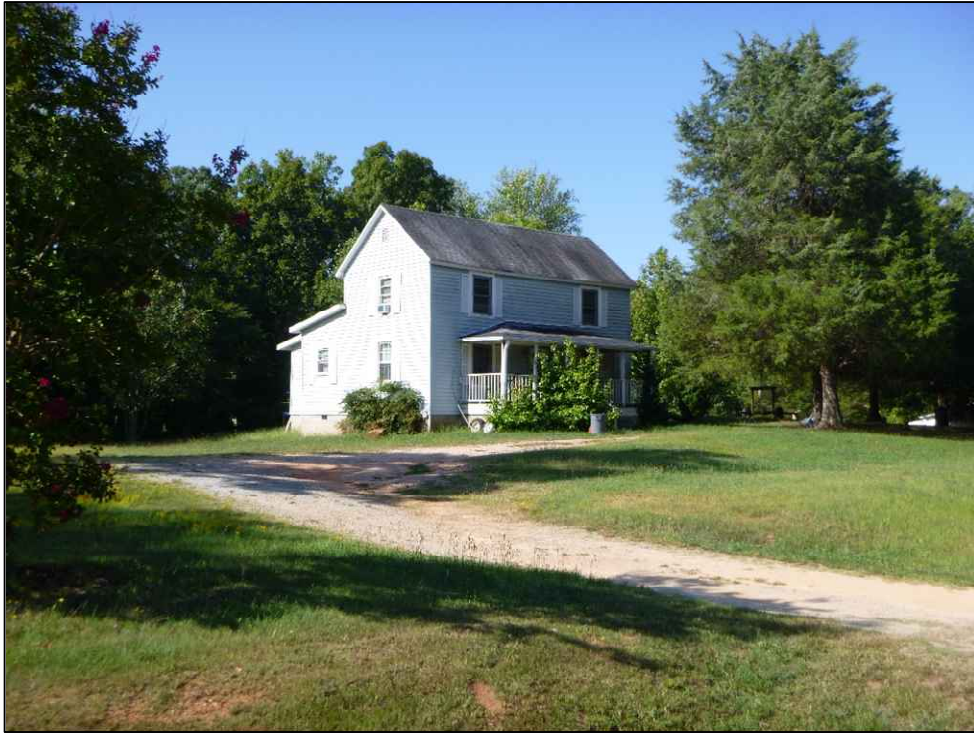
Figure 5.36. Structure 1463, facing southwest.
