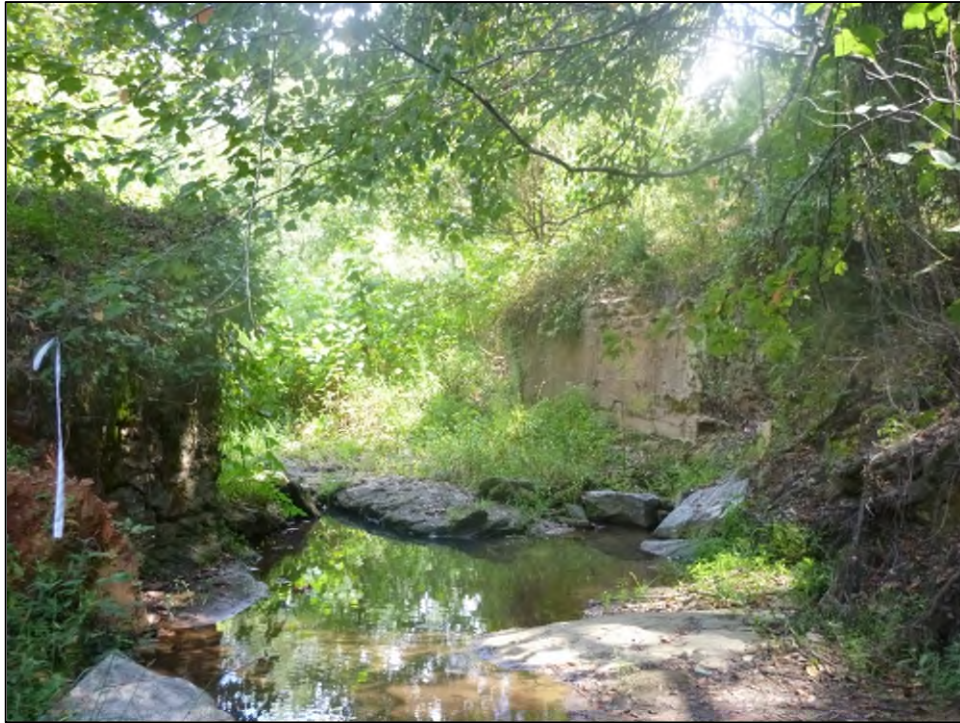
Figure 5.12. Washed out bridge on Lawrence Road in southern portion of project area, facing southeast.
