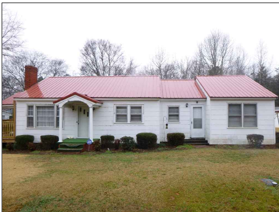
Figure 5.29. SHPO Survey Number 1653, facing north.
