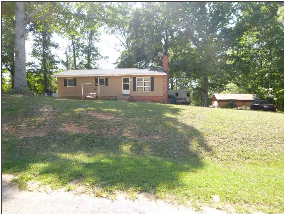
Figure 5.37. Structure 1464, facing north.
