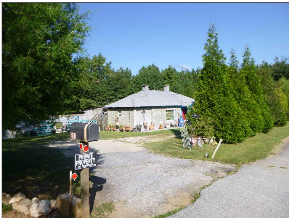
Figure 5.29. Structure 1459, facing north.
