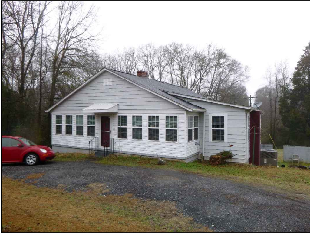
Figure 5.37. SHPO Survey Number 1661, facing north.
