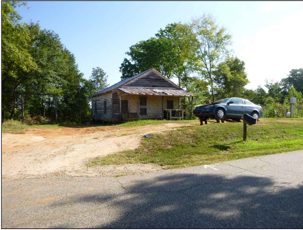
Figure 5.30. Structure 1460, facing north.
