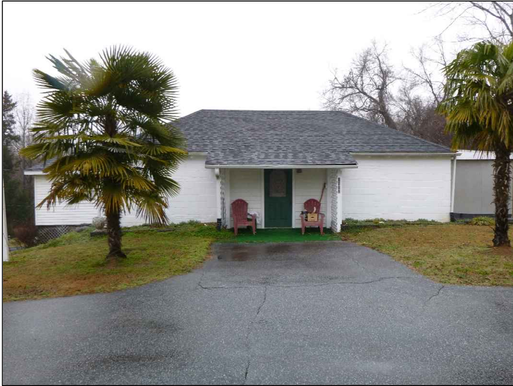
Figure 5.36. SHPO Survey Number 1660, facing north.
