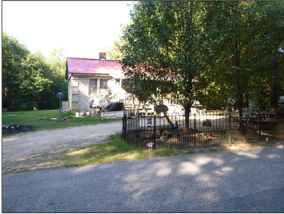
Figure 5.28. Structure 1458, facing north.
