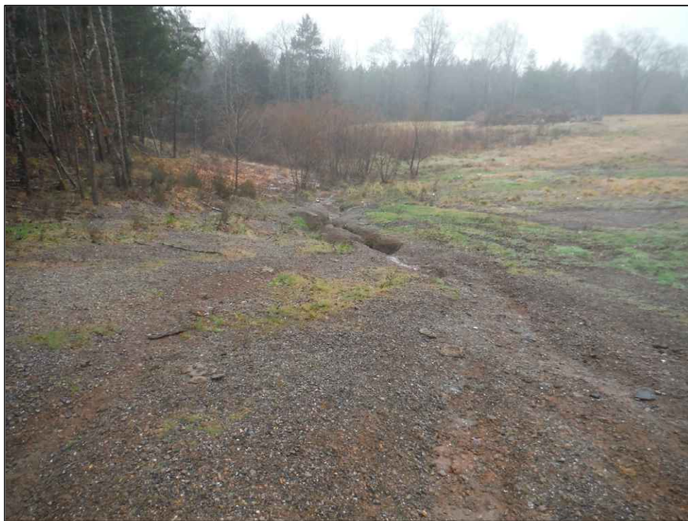
Figure 5.9. Erosion in the northern parcel, facing west.
