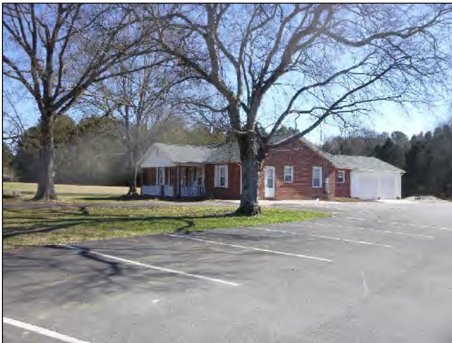
Figure 5.34. Orr Baptist Church Pastorium (0023.2), facing east.
