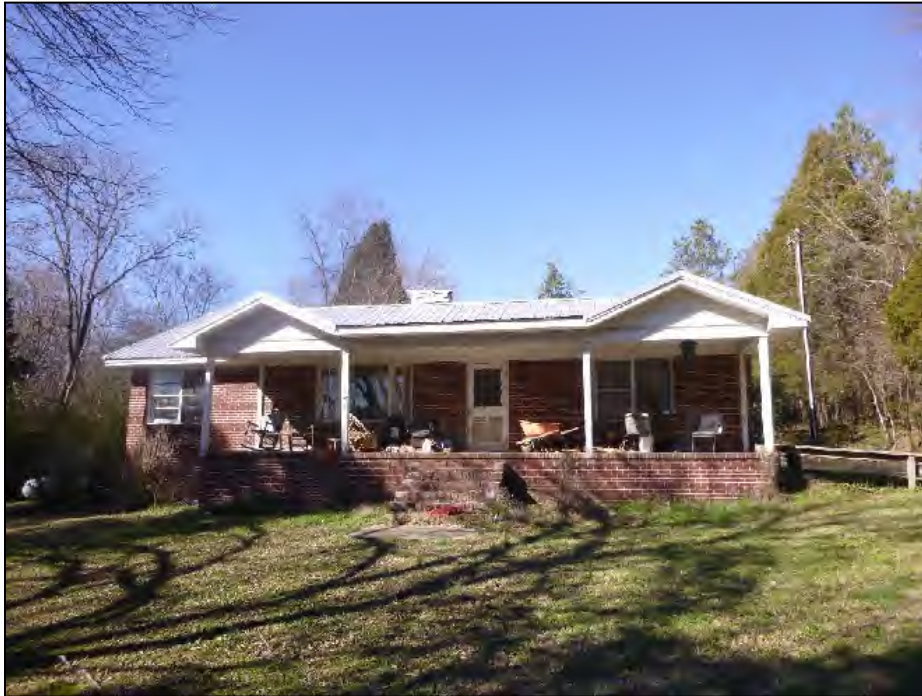
Figure 5.37. Structure 0301, facing north.
