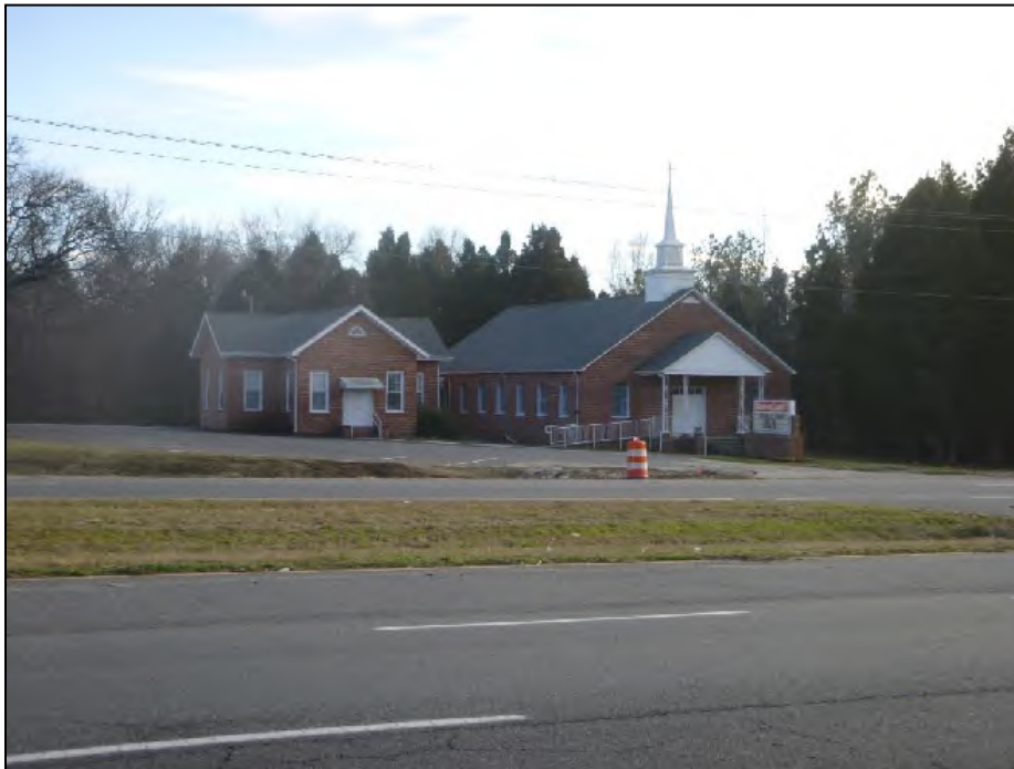
Figure 5.32. Orr Baptist Church (0023) and Chapel (0023.1), facing southwest.
