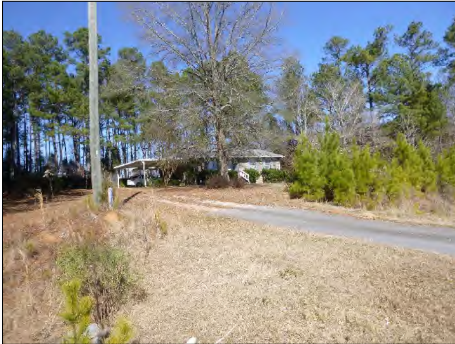
Figure 5.35. Structure 0299, facing northeast.
