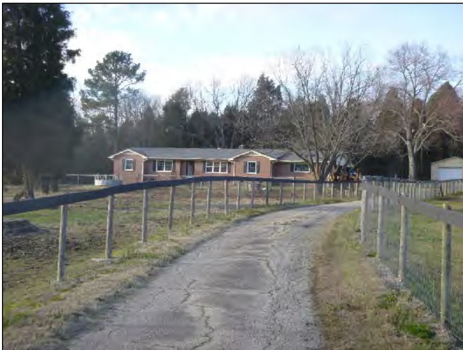
Figure 5.40. Structure 0302, facing north.
