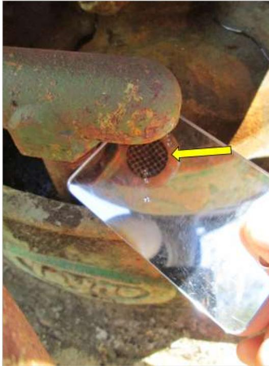
**FIGURE 5. East Voorhees well vent (well vent with screen mesh larger than #24).**
