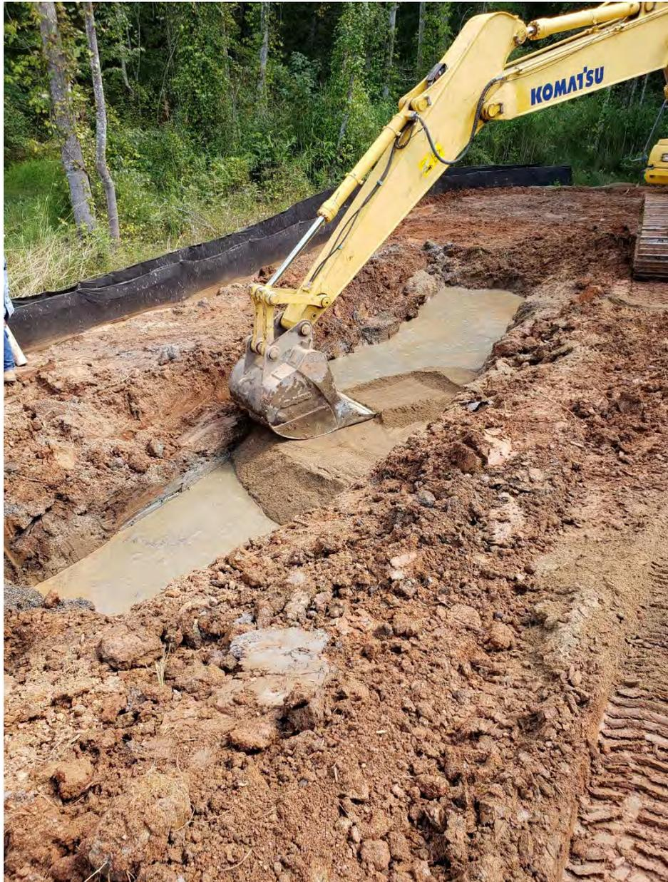
**Photograph 8: Compacting backfill with excavator.**
