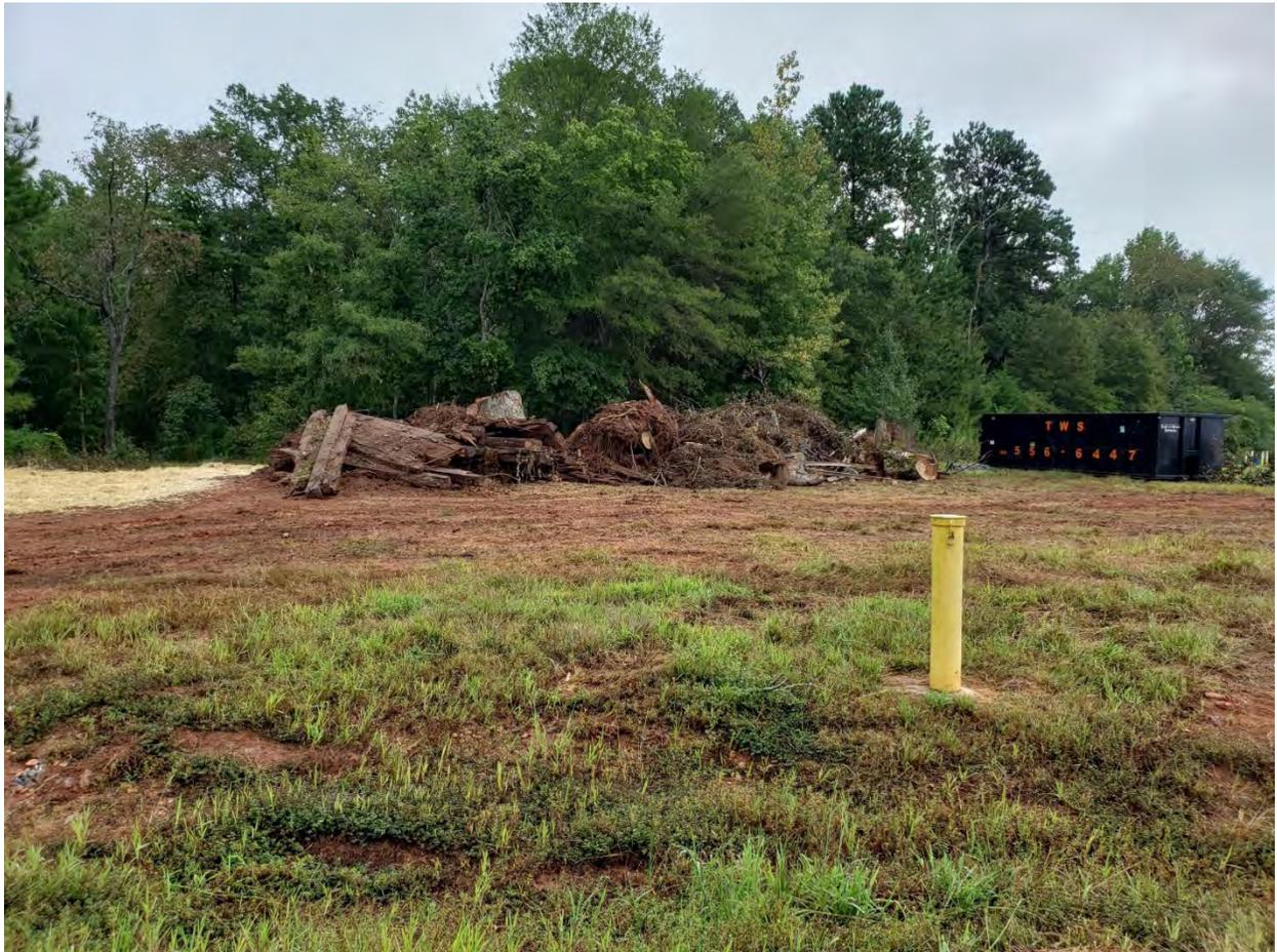
**Photograph 14: Removed timber mats and woody debris staged at stockpile area at top of hillside. Recovery well RW-5 in foreground.**
