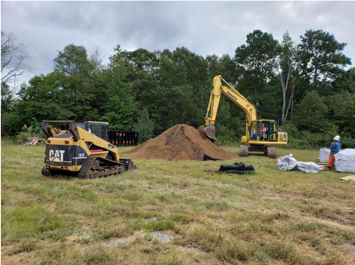
Photograph 6: Mixing sand and carbon at stockpile area.
