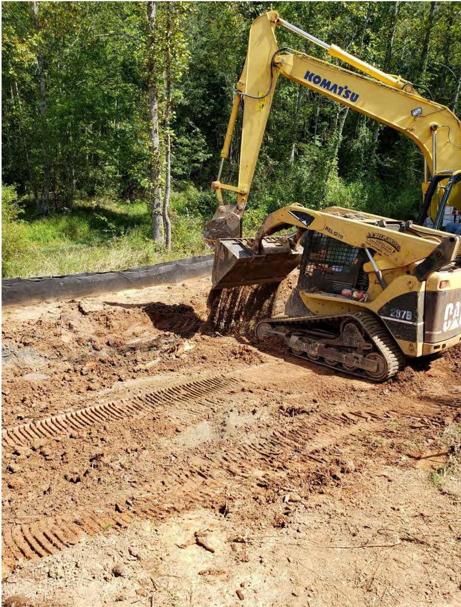
Photograph 7: Backfilling with sand and carbon mix.
