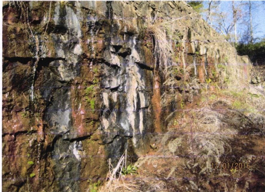
10. Closer view of the seepage and ochre along the left face
