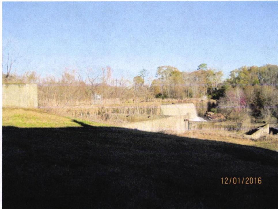
1. Overall view of the dam
