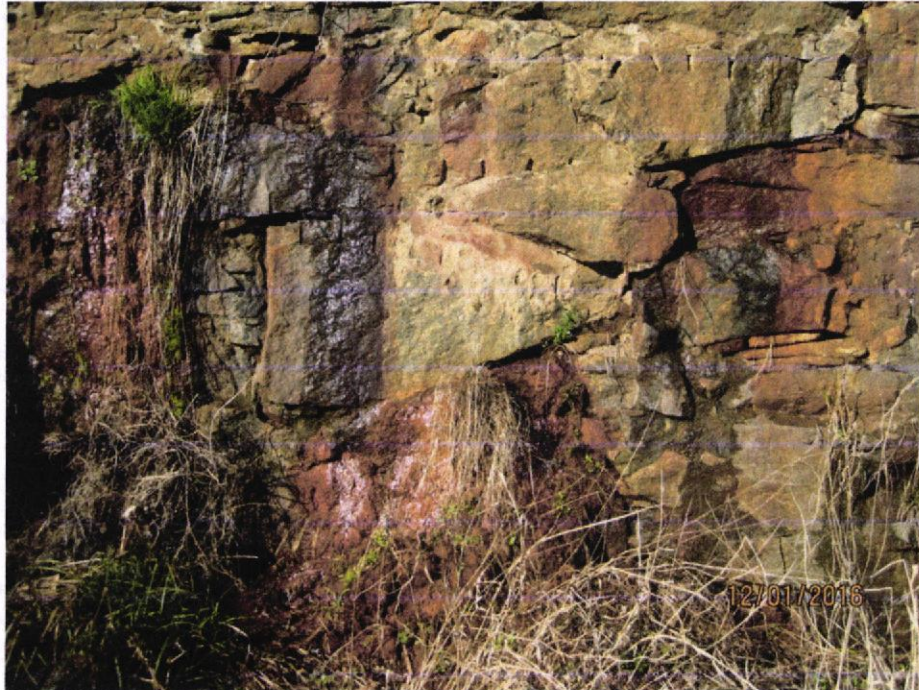
4. Closer look at the seepage and ochre present on the right face
