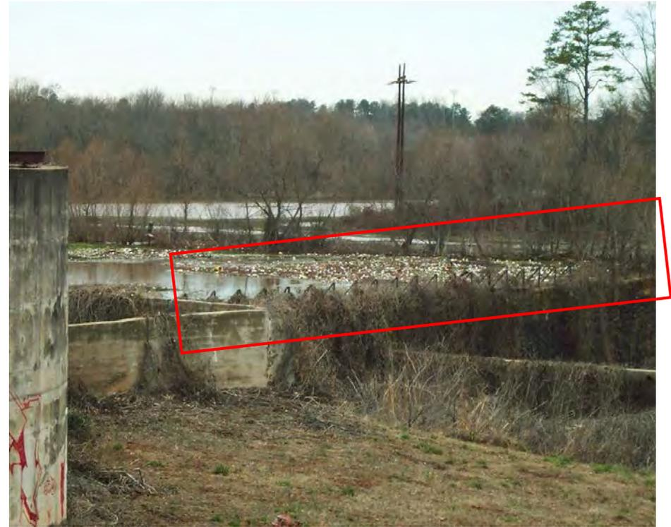
Photo 4.4: 2002. Note flashboard steel support frames.
