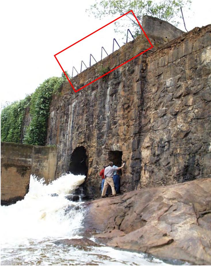
Photo 4.3: 2001. Note flashboard steel support frames.
