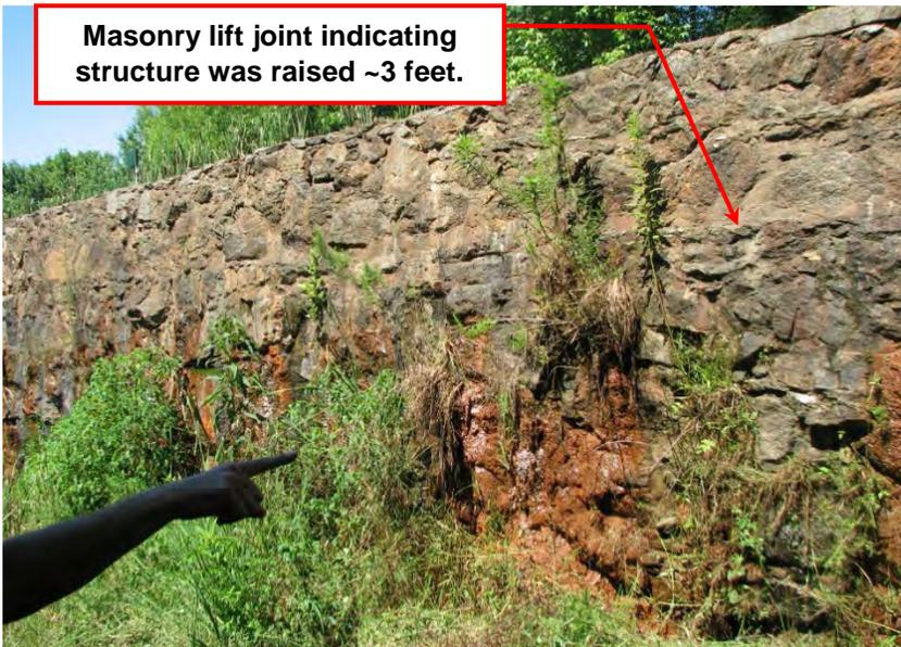
Photo 28: Left Non-Overflow Structure, seepage through dam.
