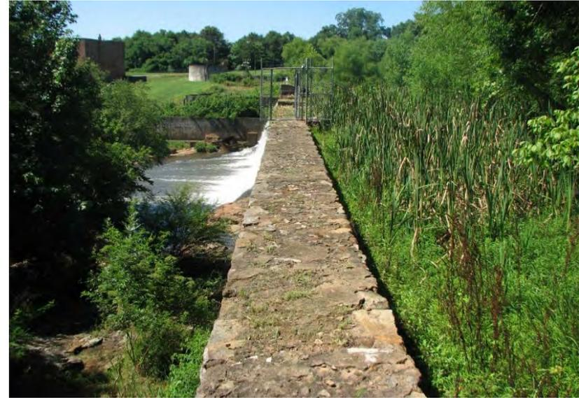
Photo 27: Left non-overflow crest; note high cattails on upstream side.
