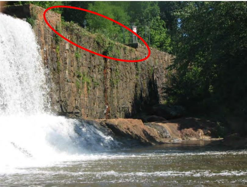
Photo 20: Spillway (circled, high crested section) and Left non-overflow beyond.
