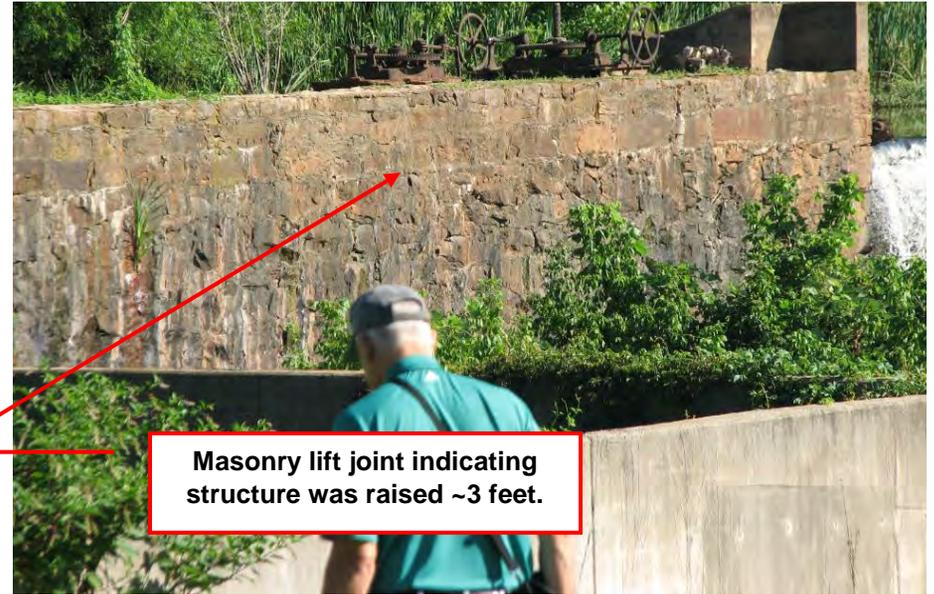
Photo 6: Right Non-Overflow; downstream side left third.
