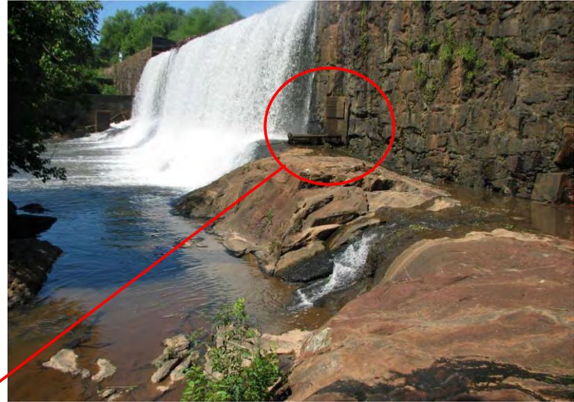
Photo 23: High crest section of spillway looking right, rock shelf along base of structure and plugged outlet gate.
