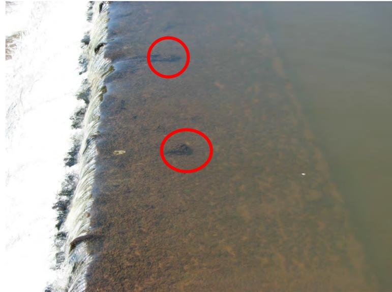
Photo 17: Spillway dam, low crest section looking right. Note remains of flashboard pins/anchors.
