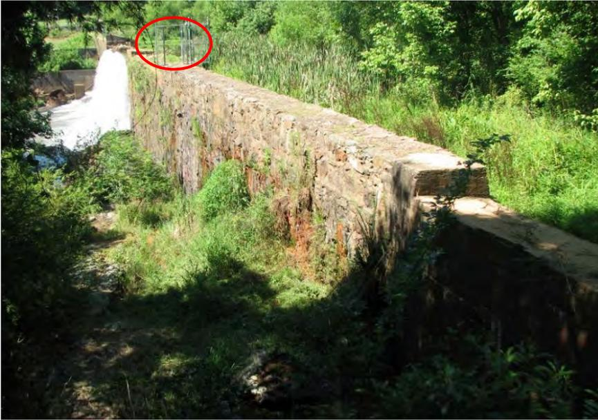
Photo 26: Left non-over flow with high crest spillway starting at fence (circled).
