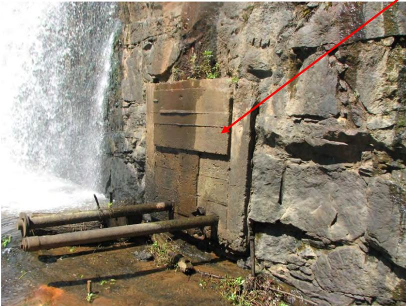
Photo 24: High crest section of spillway, plugged outlet gate.
