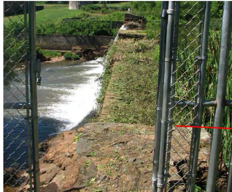
Photo 25: Looking right at dam spillway, high crest starting at red line.
