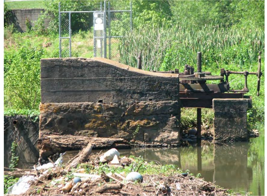
Photo 13: Outlet structure as seen from left side of spillway dam.
