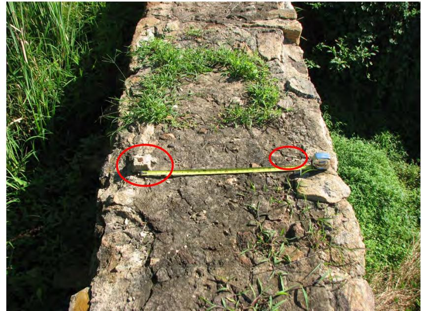
Photo 8: Right Non-Overflow, crest. Flashboard support frame anchors are circled; 2'-4" apart and spaced at 5'-3".
