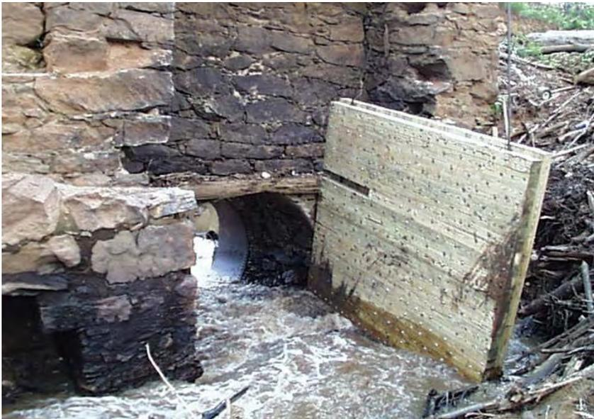
Photo13.1: June 2001, wood bulkhead installed on upstream side of intake to penstock.
