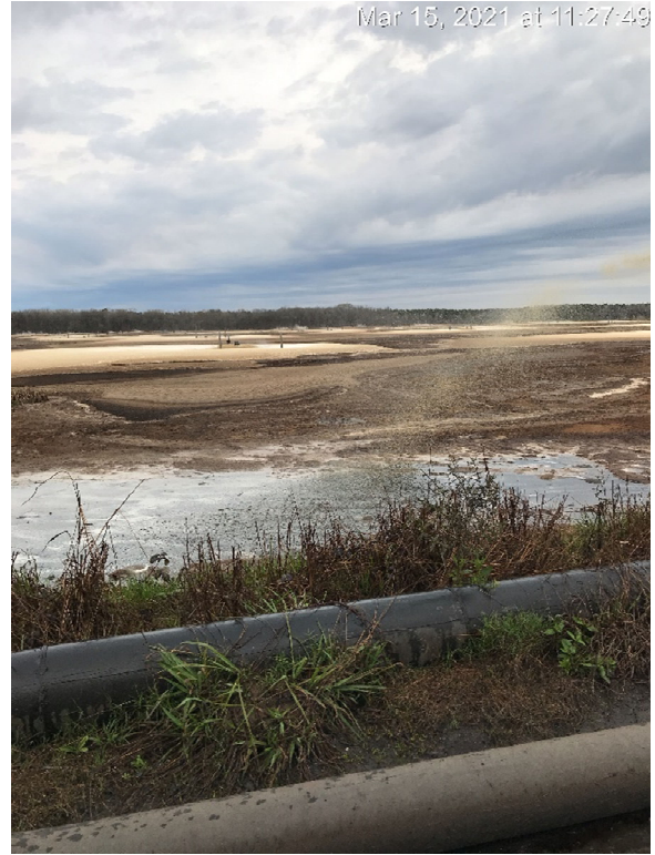
Photo ID: 4 Date/Time: 3/15/2021; 1127 Description: Aeration basin with foam layer
