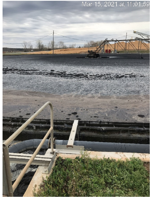
Photo ID: 2 Date/Time: 3/15/2021; 1101 Description: Primary clarifier with ash layer
