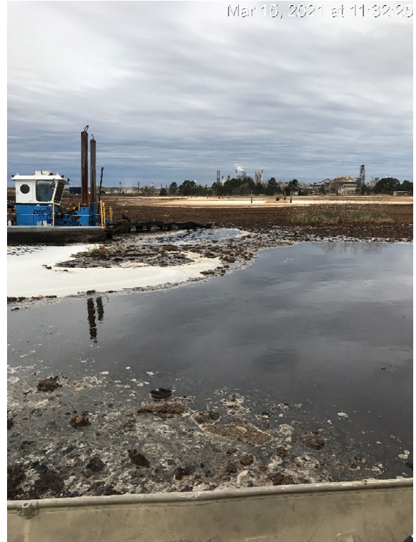
Photo ID: 6 Date/Time: 3/15/2021; 1132 Description: Dredging barge in aeration basin
