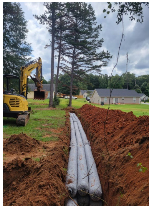
Drainfield being repaired with the installation of E7 Flow drainage lines
