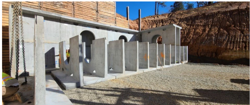
BMP6A initial vault sections installation
