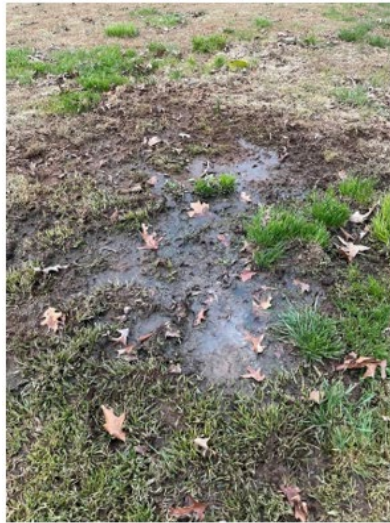
Images of a failing septic drainage field (left) and surfacing wastewater (right) in the South Tyger River Watershed
