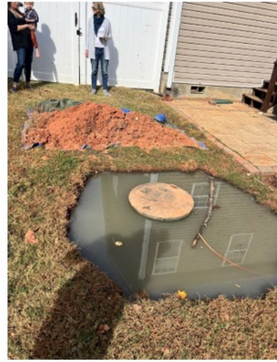
Images of a failing septic drainage field (left) and surfacing wastewater (right) in the South Tyger River Watershed
