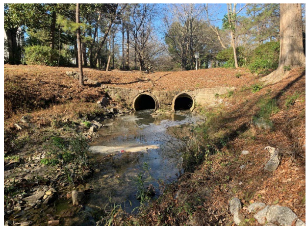
Culverts to be daylighted in the upcoming work
