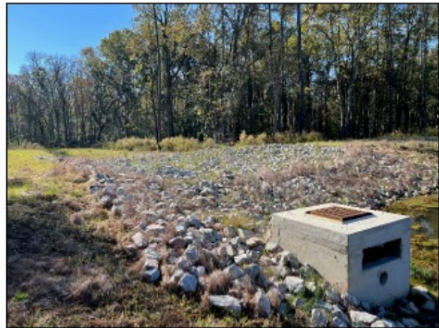
Constructed wet detention pond at the outfall structure
