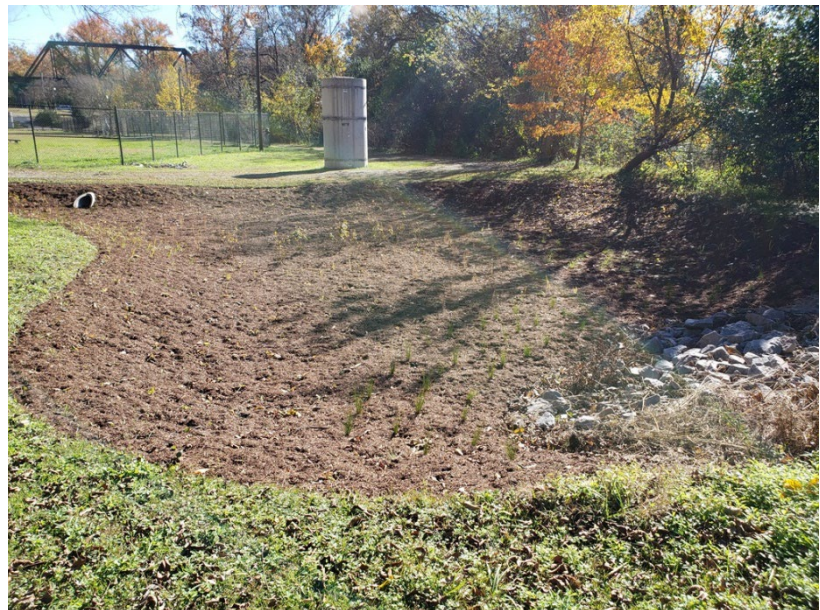
Earlewood Park bioretention area
