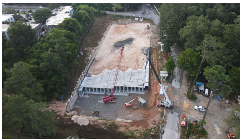
BMP6 Vault Installation
