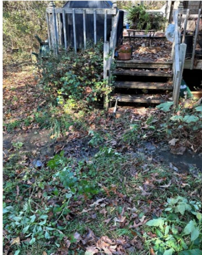
Images of failing drainage field (left) and surfacing wastewater (right) in the Three and Twenty Creek Watershed.
