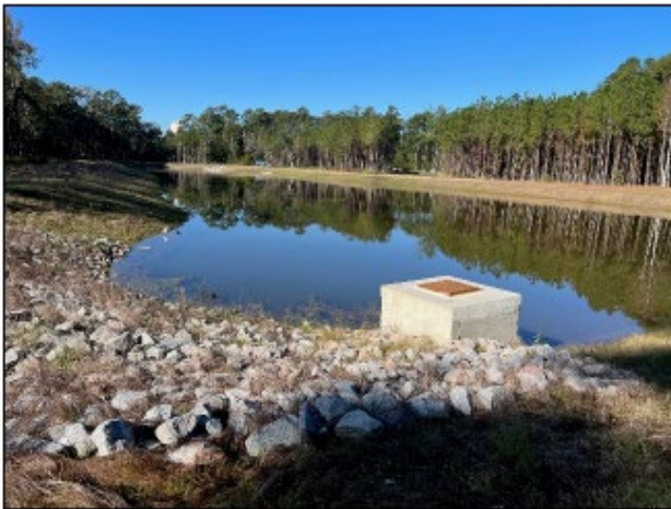
Constructed wet detention pond at the outfall structure
