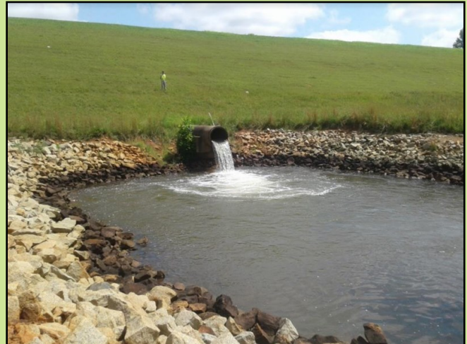
Outlet conduit and plunge pool of a regulated dam
